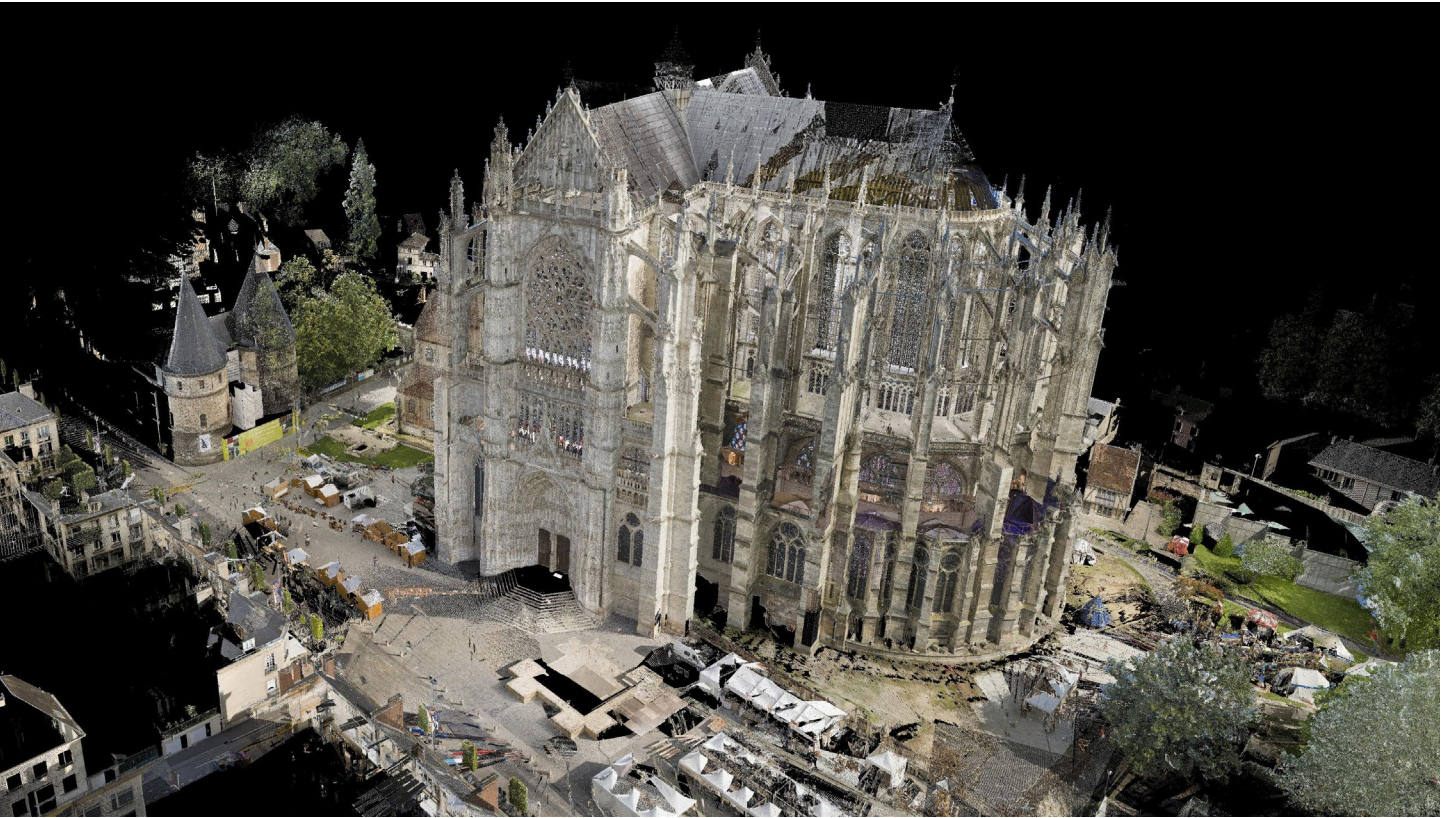
A colorized point cloud of Beauvais Cathedral in northern France.
