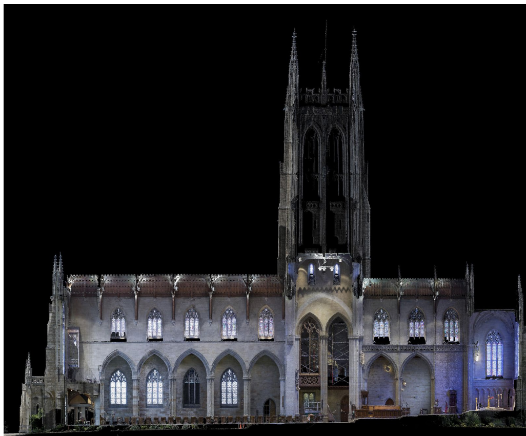
A colored point cloud of the north elevation of Bryn Athyn Cathedral.
